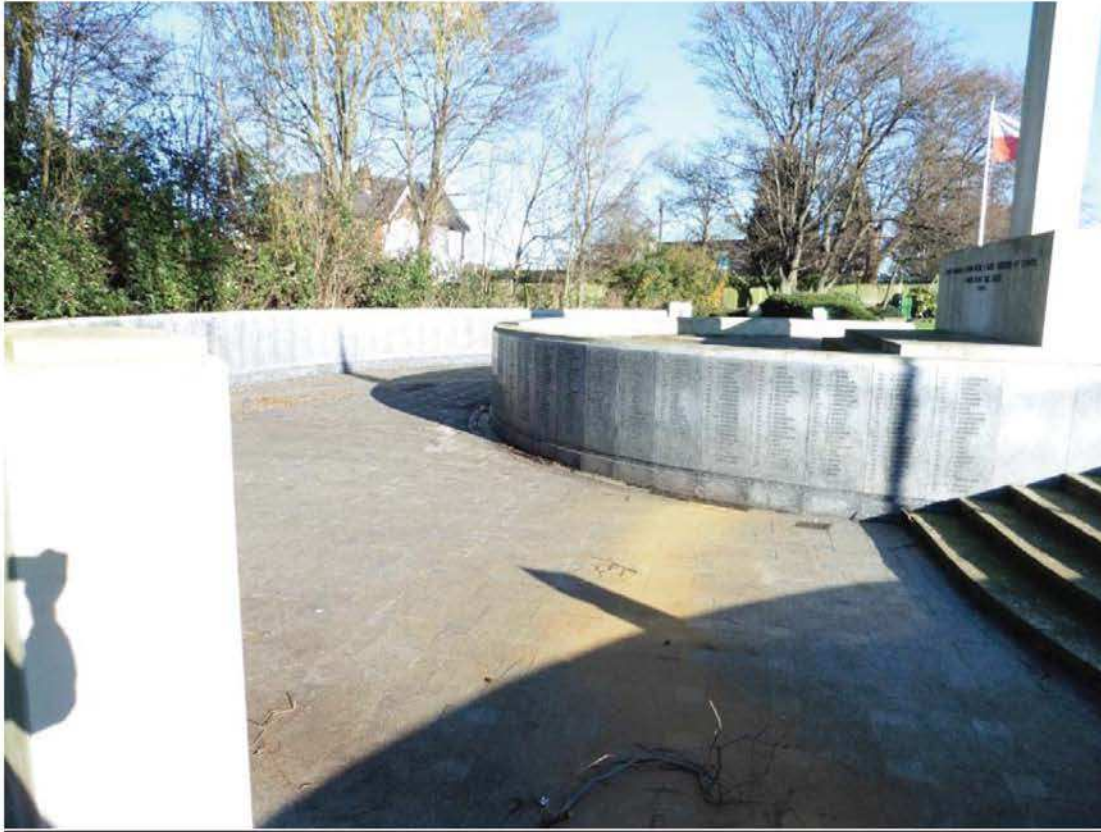
Picture 3. Showing granite paving with run off from path to remembrance garden
