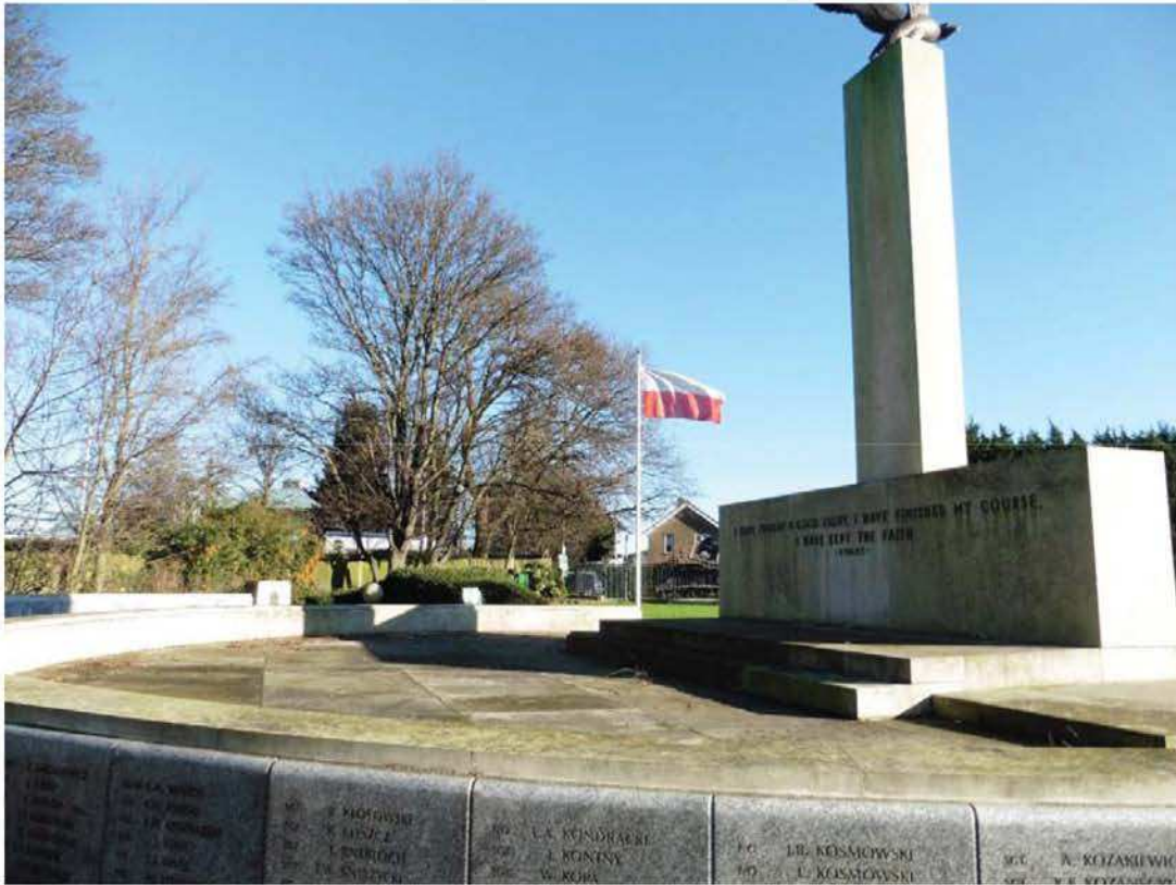
Picture 9. Portland paving and back of memorial showing signs of ageing and algal growth
